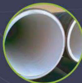
Inspection of pipes with internal cement coating from the inside of the pipe
