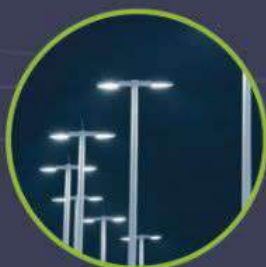
Corrosion detection in metal supports of street lights
